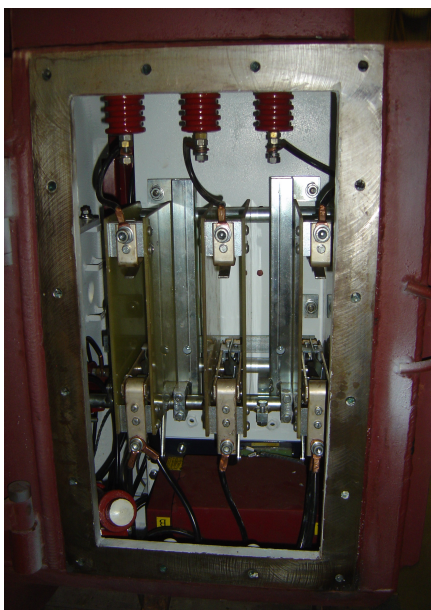
View of the GN chamber - side of the switch disconnector
